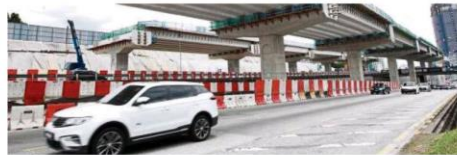
A stop-work order was issued at a SUE construction site along the MRR2 following an incident where a concrete slab fell on a car on Sept 19. — Filepic
