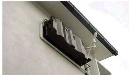
To get rebate on assessment, homeowners can instal rain harvesting system like this one. — Filepic
